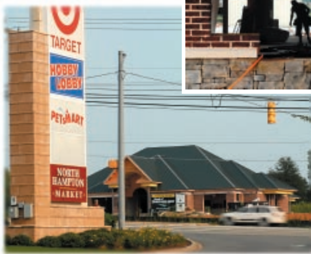
Across from Target at North Hampton Market, the construction schedule for the Wade Hampton Office is "on target," according to Paul Harper, Project Manager for Reece Construction.
